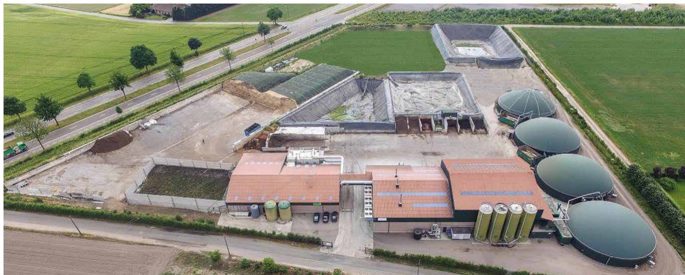
Site Biogas Bree
